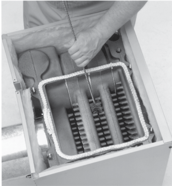
Figure 25 Thoroughly clean flue ways between all pins at all angles. Start on top of boiler, finish from the bottom.
