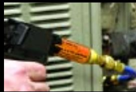
STEP 4: CLEAN PORT & DISCARD EMPTY CARTRIDGE
