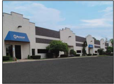
European Sales Office and Warehouse
