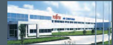
Fujitsu General (Shanghai) Co., Ltd.
