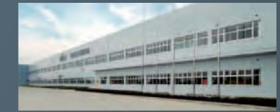
Fujitsu General Central Air-conditioner (Wuxi) Co., Ltd.
