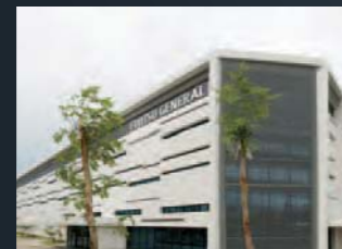
R&D Center in Fujitsu General Engineering (Thailand)
