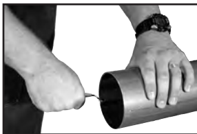
Figure 3: Deburr inside diameter deburring tool
