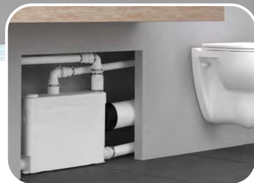
View of installation behind the wall
