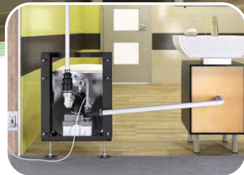
View of installation behind the wall
