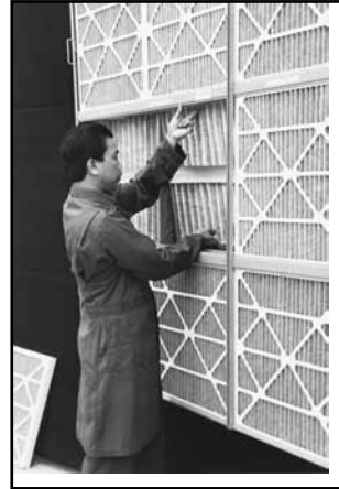
Installing filters and prefilters
