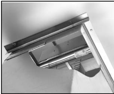
Through Ceiling Membrane Penetration
