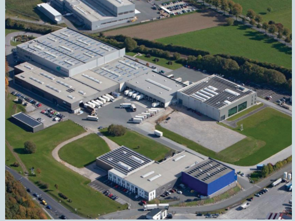
Centrotherm Systemtechnik GmbH Brilon, Germany
