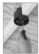
Just one hand is required to mount the box using the pre-located mounting screw.
