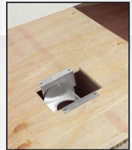
Mount SureGrip support plate.
