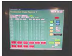
Computer Automated Duct Line Controller
