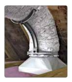
Flexible duct is often susceptible to kinks and sags that restrict air flow. The FDS1 Flexible Duct Support eliminates air flow restrictions and increases efficiency to dramatically reduce utility bills and improve heated or air-conditioned room comfort. A properly supported 90°duct elbow typically improves air flow efficiency 10 to 40%. A Malco Duct Support quickly installs on new
