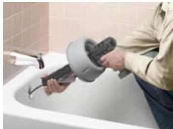
K-39AF quickly opens clogged tub lines.
