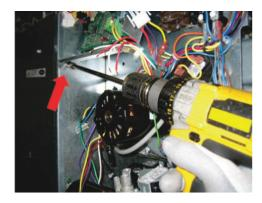
Fig. 34 – Removing Screw Under Control Board Panel A2100/8
