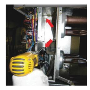
Fig. 33 – Removing Screws Behind Heat Shield
