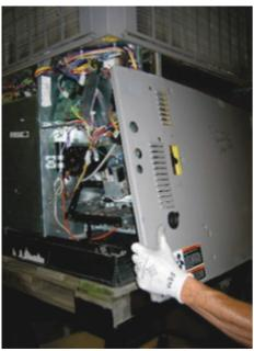
Fig. 37 - Replacing Right Side Panel
