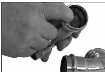
Figure 2 — Check for EPDM Seal
