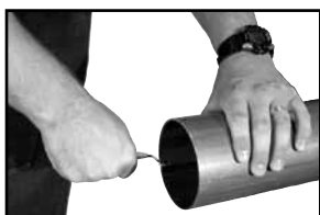
Figure 3: Deburr inside diameter deburring tool
