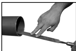
Figure 2: Deburr inside diameter using a half-round file
