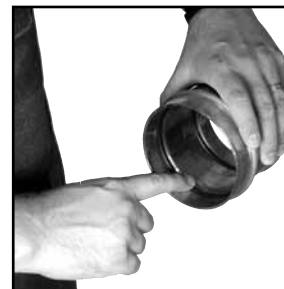
Figure 5: Check for EPDM seal
