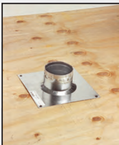
Push pipe through vent support.
