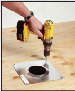
Mount SureGrip support plate.
