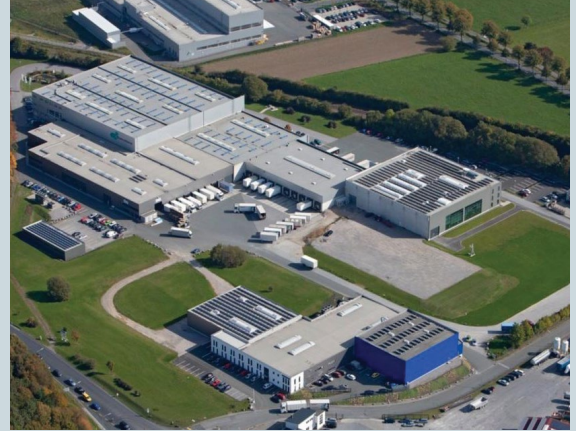
Centrotherm Systemtechnik GmbH Brilon, Germany
