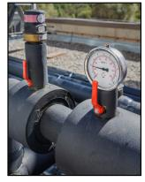
expected, AEROFLEX should be protected with a jacketing system.
