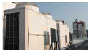
Traditional VRF top-discharge outdoor units
