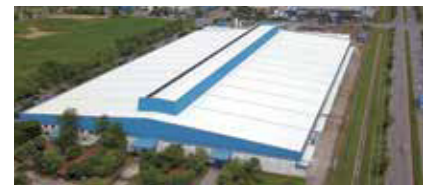
Fujitsu General (Thailand) Co., Ltd. (Thailand) FACTORY-2
