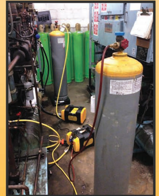
Below: On a R407a system retrofit of a low temperature ice cream case, the G5Twin recovered 600lbs of R22 in record time using the Push-Pull Method .
