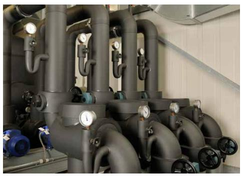
Armacell's newest innovation, ArmaFlex Ultra with FlameDefense<sup>™</sup> Technology, is the **first** elastomeric foam insulation Classified by UL to UL 723 at 25/50. This third-party certification proves our commitment to product safety and compliance. All AP ArmaFlex-branded products are made with Microban<sup>®</sup> antimicrobial protection, are GREENGUARD Gold certified and now have Environmental Product Declarations (EPDs) to show our dedication to material transparency.
