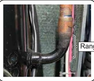
20. Cut the discharge pipe in this range.
