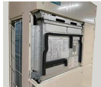
1. Remove the 4 mounting screws.
