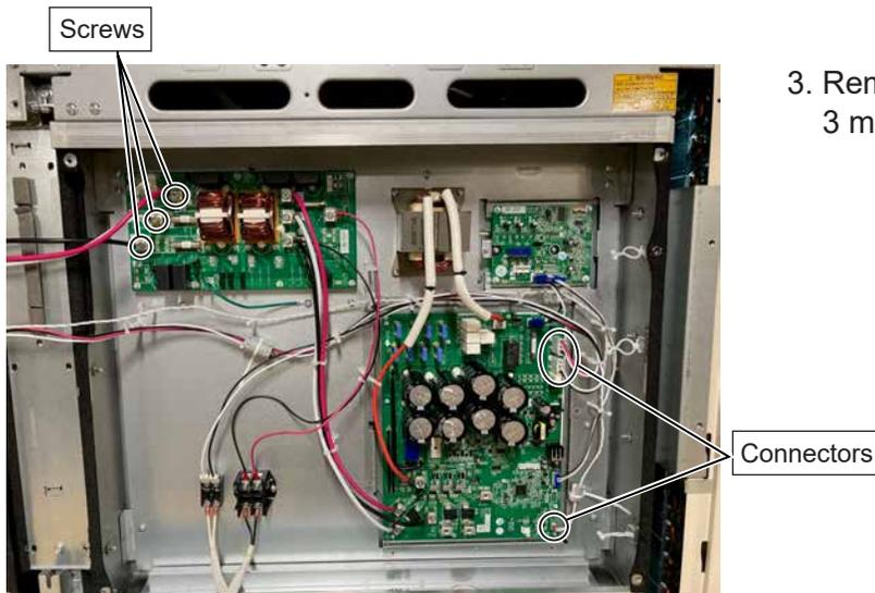
3. Remove the connectors, cables, 3 mounting screws and cable ties.
