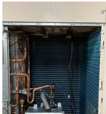
4. Remove the CONTROL BOX R by sliding upward.
