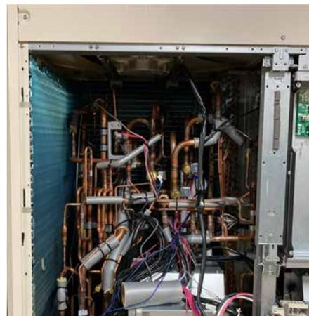
5. Remove the CONTROL BOX L by sliding upward.
