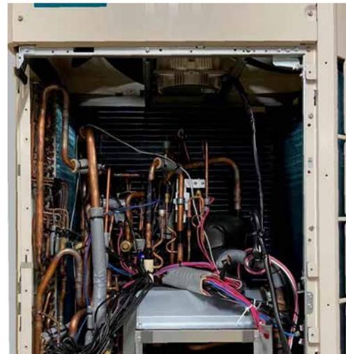
5. Remove the CONTROL BOX by sliding upward.
