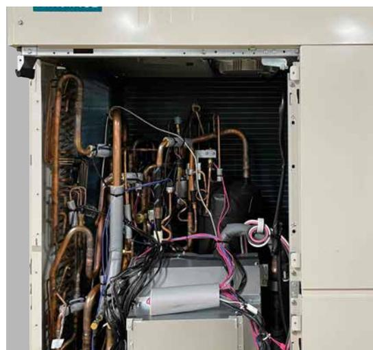
5. Remove the CONTROL BOX by sliding upward.
