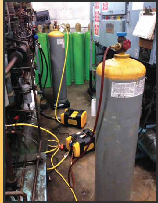
Below: On a R407a system retrofit of a low temperature ice cream case, the G5Twin recovered 600lbs of R22 in record time using the Push-Pull Method
