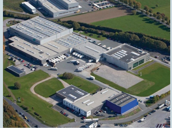
Centrotherm Systemtechnik GmbH Brilon, Germany
